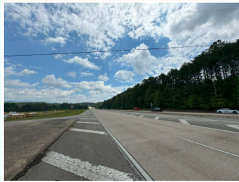
View of W. Hwy 515 Looking East
